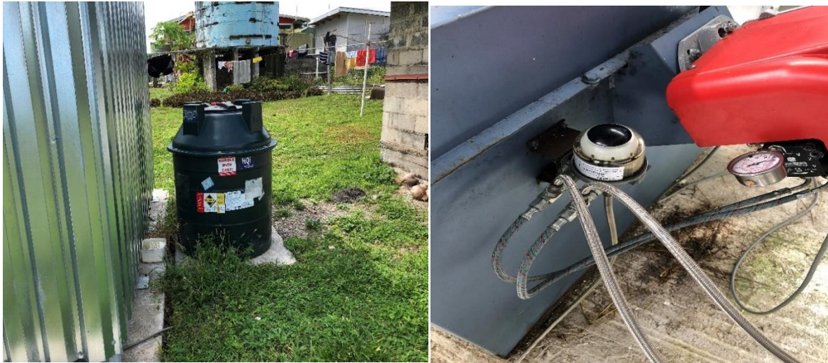
Ground mounted fuel tank and dearation device on Inciner8 i8-75a.
