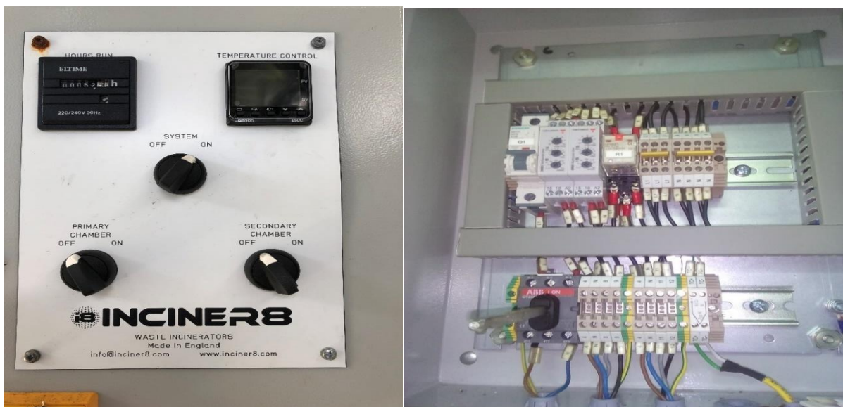
Inciner8 i8-75a control panel. External and internal Views.
