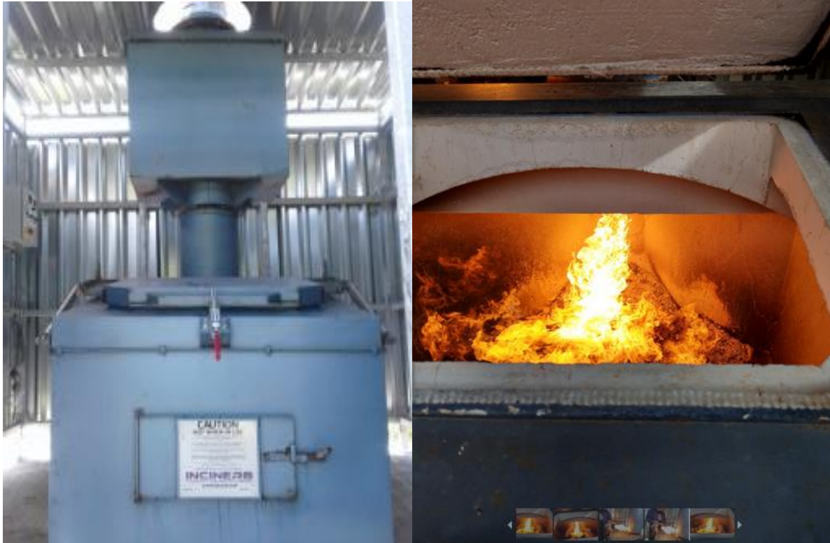
Inciner8 i8-75a primary and secondary combustion chambers
