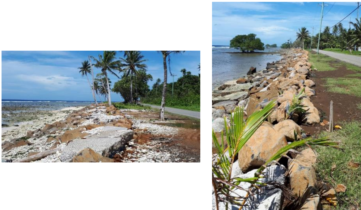
Figure 11: Existing emergency coastal defence works at Mosral (left) and Paal (right)
