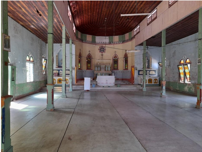
Figure 18. PACM use in church internal wall (above the concrete wall)
