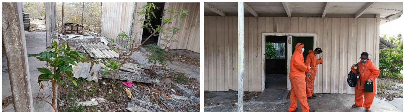
Figure 3. Look ACM roof near the outpatient building which believed to have come off from main building
