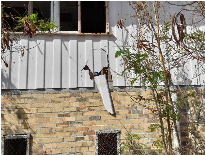
Figure 13. Broken exterior wall cladding at double storey - JSS
