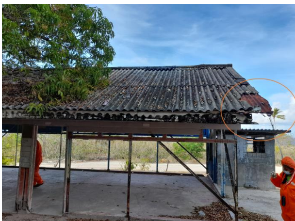
Figure 10. Former Class from with broken roof at the end; replace with aluminum roof as circled in red
